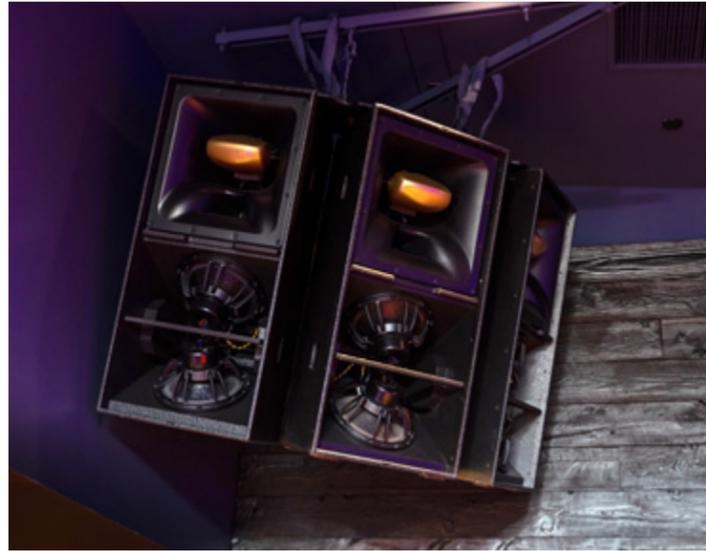
Among the products, the team utilized 12 of the XY-2E which allows the venue to build point-source arrays in a wide variety of configurations. The XY-2E maintains the favored X-phase system while enabling individual control of the 8-inch cone driver and 1-inch compression driver.
