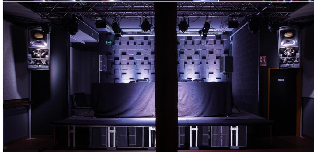
Services installed a four-point system with XY-3B three-way full range speakers either side of the stage, XY-2 mid-high speakers at the rear of the room and a trio of XY-218HS dual 18-inch horn-loaded subwoofers supplying powerful low-end. Using presets on the mixer, the club's management can easily switch to a live gig configuration which uses only the boxes at the front.
